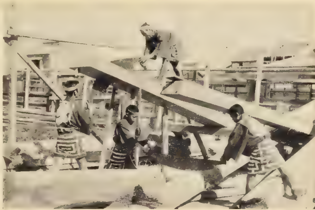
CARPENTERS AT WORK.
